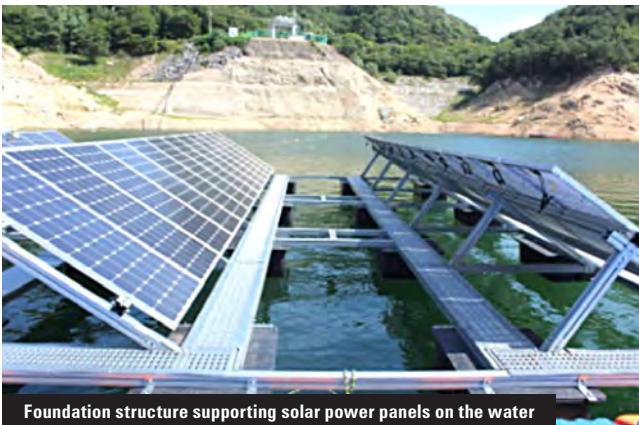
Foundation structure supporting solar power panels
